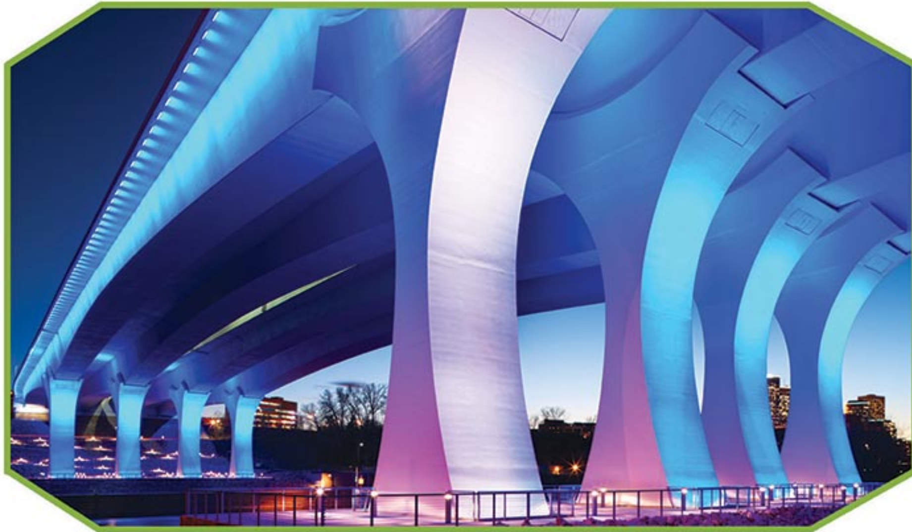
Concrete Segmental Bridges
