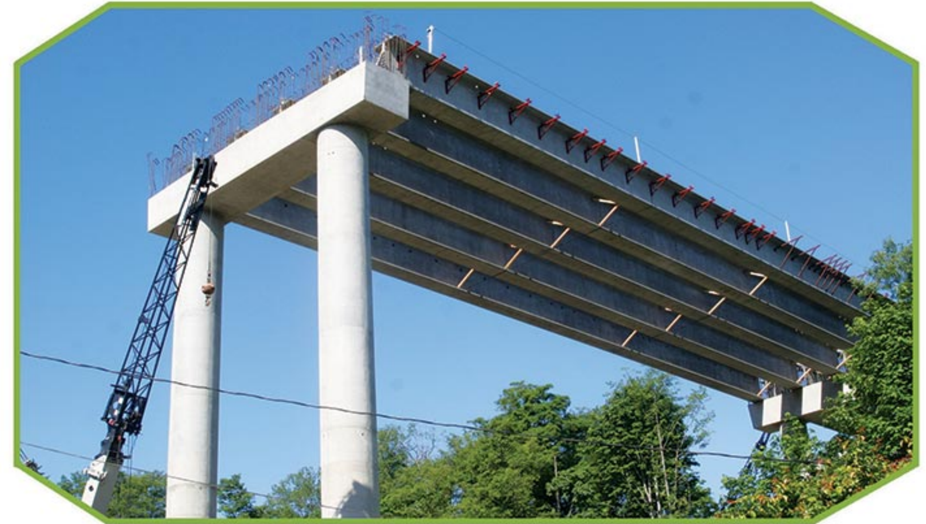
Concrete Spliced-Girder Bridges
